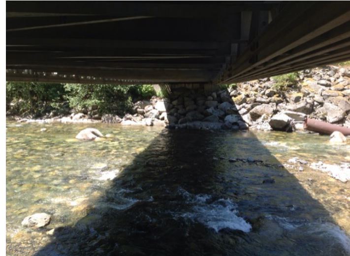
Right Bank Abutment when facing downstream
