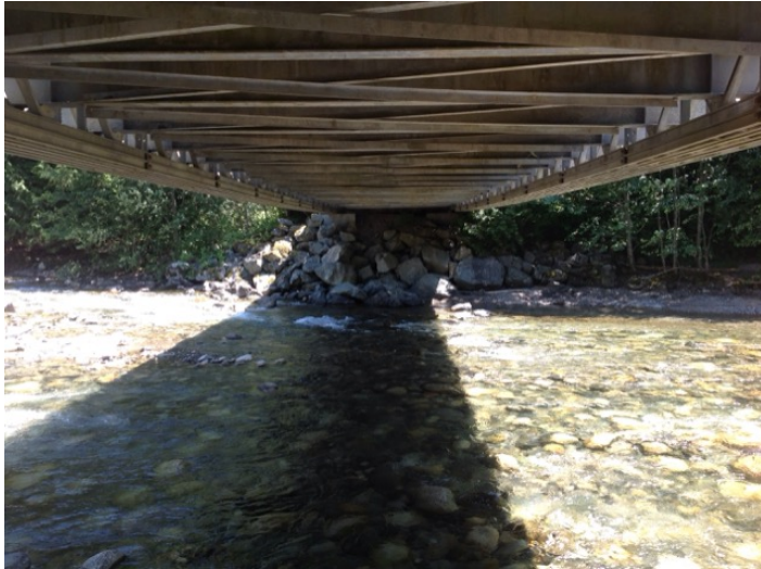
Left Bank Abutment when facing downstream
