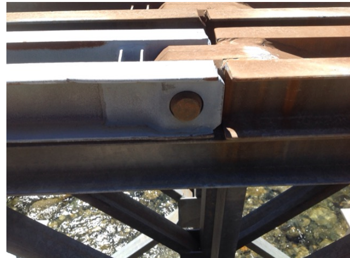
odd pin without circlip
